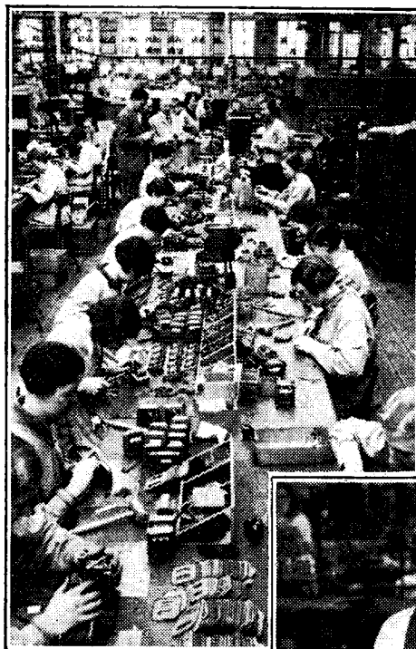
(Above) Assembling LF transformers of the AF5 and similar types.
